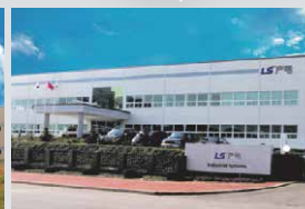
Dalian factory (China) MV/LV switchgear, MV contactor
